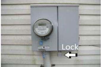
power is on but has been turned off and locked at the service disconnect. Remove any padlock before the inspection.
