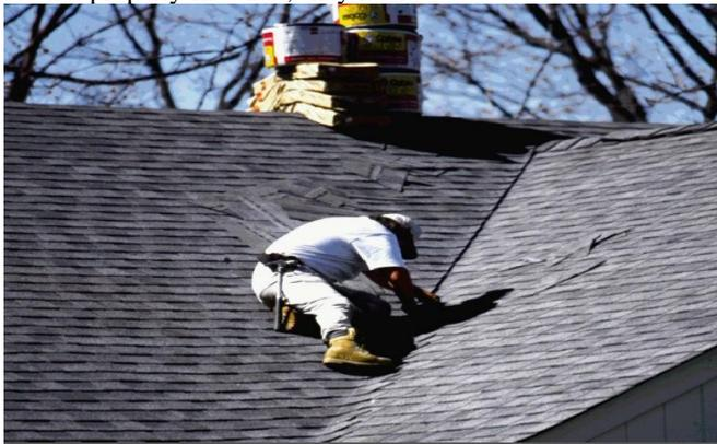
Valleys should have valley flashing installed underneath to act as a secondary barrier against leaks in case water makes it through the shingles. This is often not the case. For closed valleys (valleys covered with shingles) the flashing should consist
