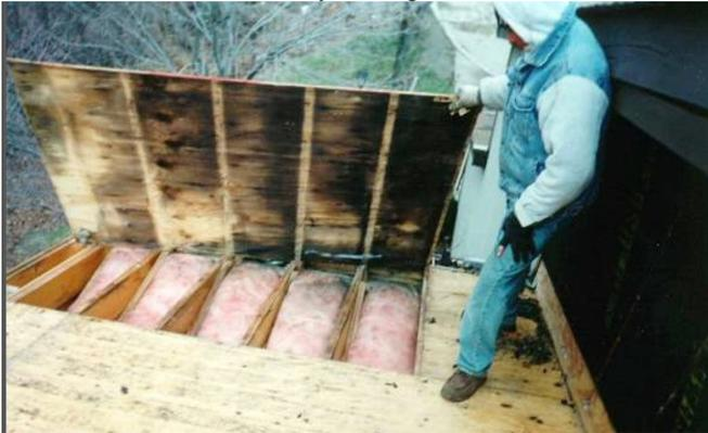
It is very common to see under ventilated attics. This is very easy to check by measuring the temperature in the attic on a hot day. If it is 140 degrees, you may want to consider increasing the amount of ventilation to help remove the excess heat.
