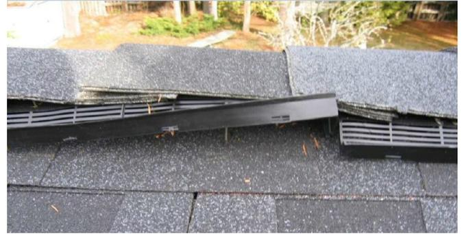
flexible and do not provide a good nailing surface for the ridge shingles. Also, sometimes the installation leaves a lot to be desired. Some roofers will cut corners and not follow the manufacturer's installation instructions. Over time, the vents can curl or twist, allowing water in.
