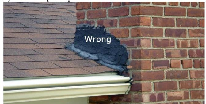
Flashing against a vertical wall must be the step flashing method. You place a shingle, and then install a piece of flashing on top of the shingle, and then repeat the process all the way up the wall. Any water running under the flashing will run on top of the shingle below and eventually into the gutter. Step flashing rarely ever leaks. Most of the time we see continuous flashing which is one long piece of flashing.
