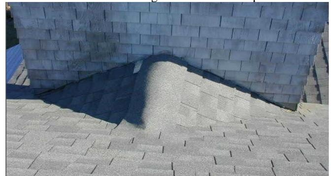
To eliminate the problem, a cricket can be installed to divert the water around the chimney. It is nothing more than a pitched section of roof that will divert the water around the chimney. This can be added to any roof when the shingles are replaced.
