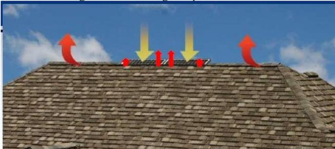
rises, it will be trapped at the highest point which is at the ridge of the attic. A ridge vent allows the heat to easily escape. As in all products on the market, there are good ones and bad ones. The good ones are rigid, and the ridge shingles can be easily nailed down the vent and designed to prevent rain from blowing into the sides and into the attic. The bad ones are
