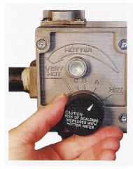
heater has an external thermostat, and an electric water heater internal has an thermostat located behind an access cover. Both controls can be set anywhere between Hot and Very Hot ." Always set the temperature of the water around 120° F. Temperatures than 125° F can burn a child or an adult quite severely and
