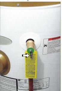
point of 212° F, and this can increase the pressure inside the tank, resulting in the heater water exploding. There have been accounts of water heaters taking off like rockets and landing several hundred feet away from the home. water heaters A11 should have a safety called device temperature and pressure release (T&P) valve. The T&P valve will sense a temperature of 210° F or a pressure of 150 psi and open, allowing
