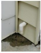
into a crawl space, the end of the pipe is not readily visible and you would not necessarily know if the valve is leaking. The most common location is outside of the house. The pipe should turn down and extend to within 6 inches of the ground or pavement.
