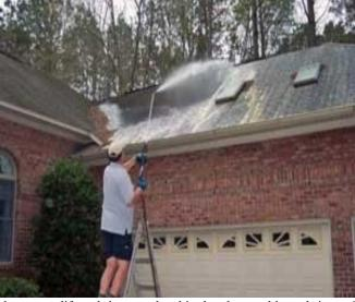
the sun or lift and damage the shingles that could result in roof leaks. If you do use a pressure washer, be sure to use very low pressure and wash from the rear of the shingle or from the ridge down to prevent blowing water under the edge of the shingle, lifting and damaging the shingle.
